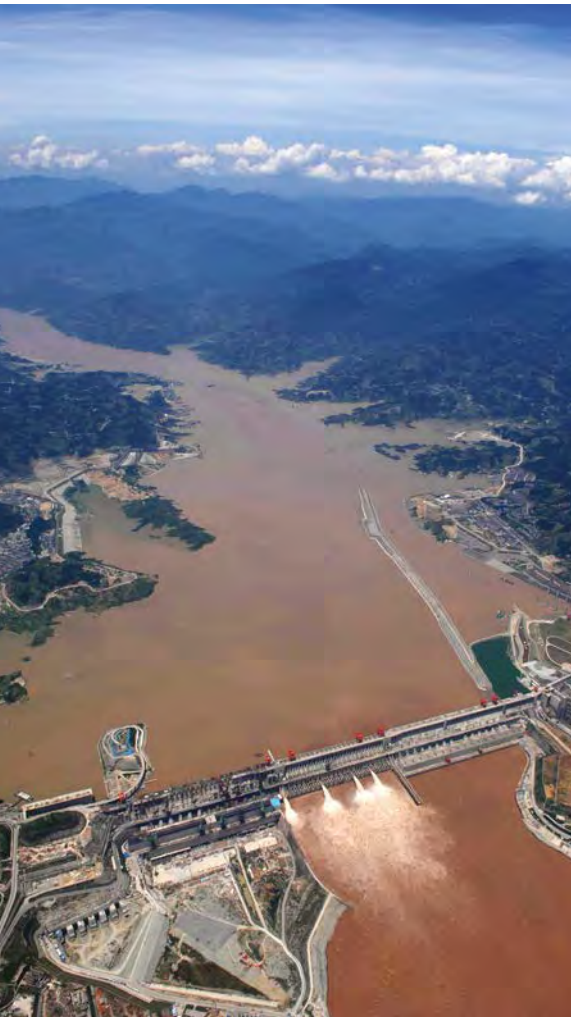
Source 3 An oblique aerial view of the Three Gorges Dam on the Yangtze River in China. Water flows through the open sluice gates. The hydroelectric power station is to the left of the sluice gates.
