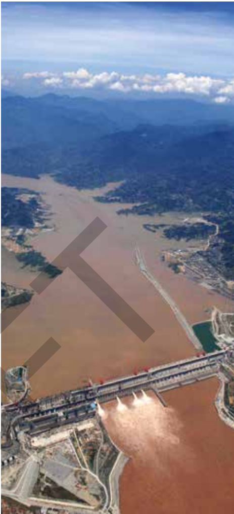
Source 3 An oblique aerial view of the Three Gorges Dam on the Yangtze River in China. Water flows through the open sluice gates. The hydroelectric power station is to the left of the sluice gates.
