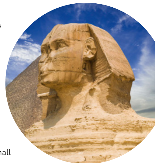
Figure 6.57 The Great Sphinx of Giza in Egypt has been badly damaged by wind erosion.
