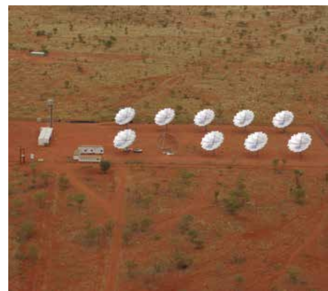
Source 4 The solar power station provides 50 per cent of daytime electricity needs to Yuendumu and enables significant reduction in the diesel fuel used in power generations in the community.
