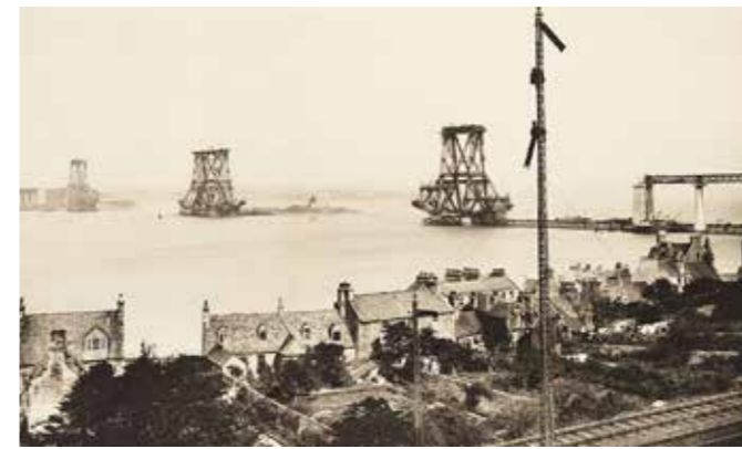
Source 8 The Forth Railway Bridge in east Scotland under construction. By the time of its completion in 1890, it was the longest bridge of its kind.
