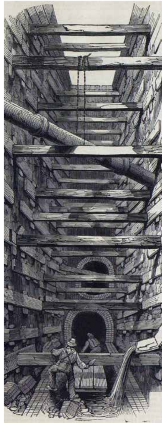
Source 1 The building of a London sewer, 1845
