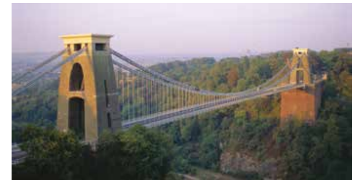
Source 3 Clifton Suspension Bridge, as it stands today in Bristol
