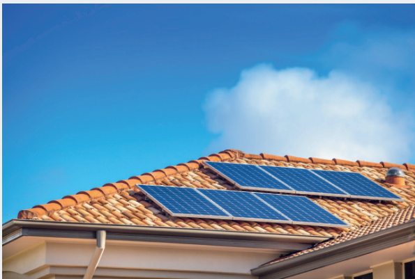
Figure 6 Solar panels improve energy efficiency.
