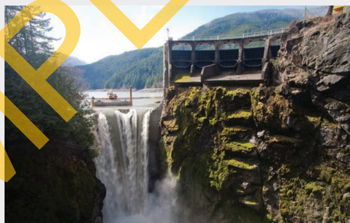
Source 1.60 The 64-metre-high Glines Canyon dam partially removed in March, 2012.
