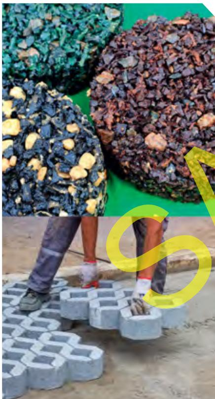
**Figure 2.40** New products have been developed that allow water to move through instead of contributing to run-off. This allows the water to be absorbed into the soil and join the groundwater.
