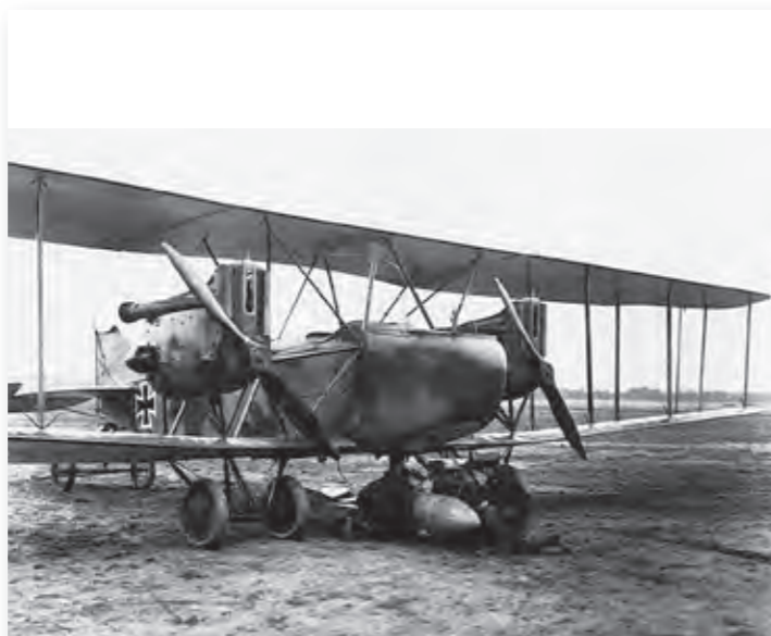
Source 5.24 German airmen attach a 100-kilogram bomb to the underside of a Gotha bomber.
