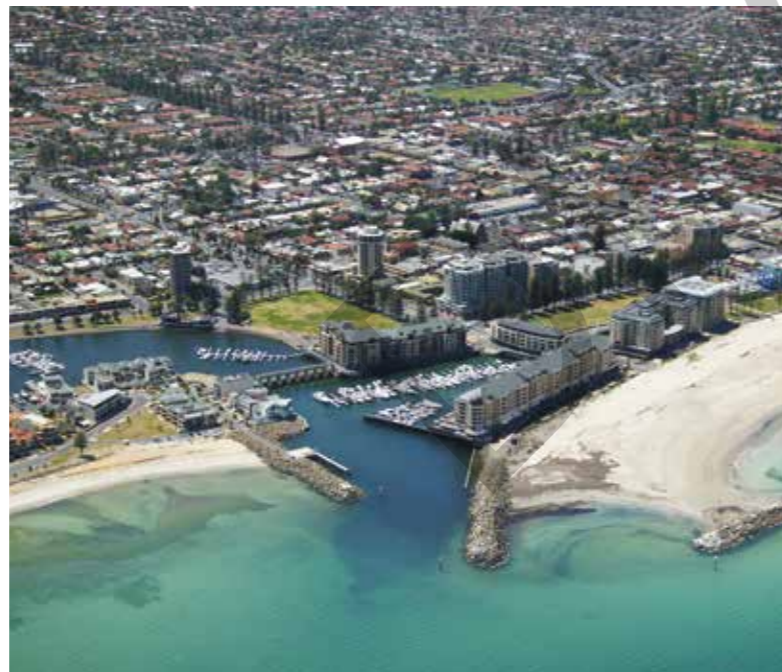
Source 2 Two training walls and a breakwater have helped to trap sand at the mouth of Glenelg Harbour in Adelaide.
