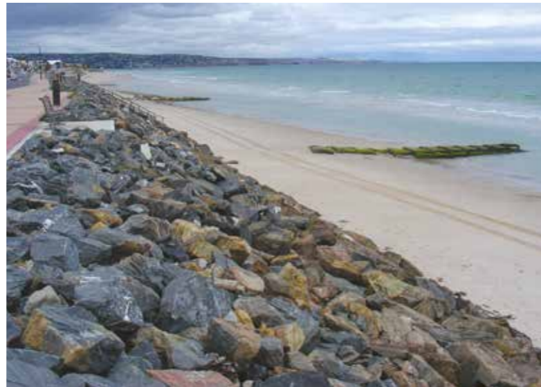
Source 1 These groynes near Brighton Beach in Adelaide were built to protect the millions of cubic metres of sand pumped onto this beach in the 1990s.
