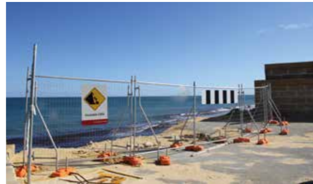
Source 1 Coastal erosion has caused a road to collapse in Seabird, Western Australia.
