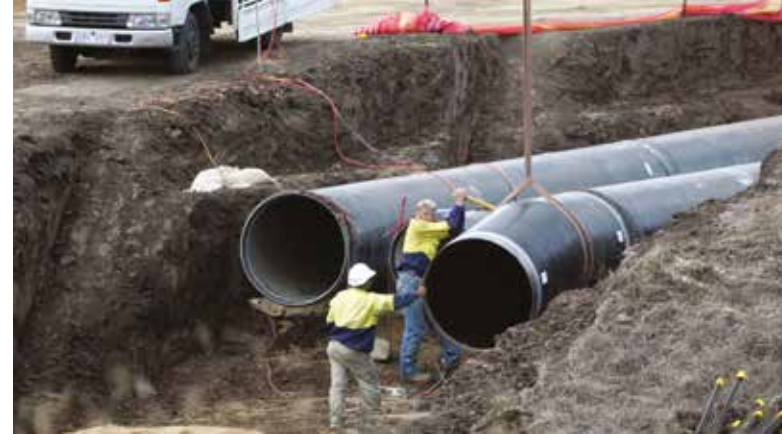
Source 4 Huge pipes carry water beneath our city streets. Here, pipes are being laid in Brisbane.
