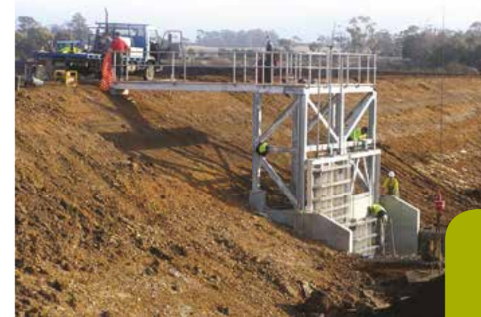
Source 4 Steel gates are installed in the levee at Longford, Tasmania.
