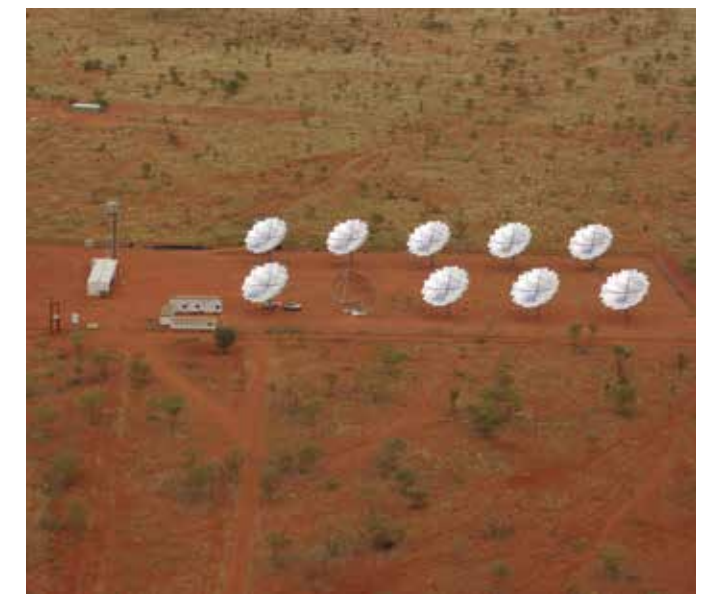
Source 4 The solar power station provides 50 per cent of daytime electricity needs to Yuendumu and enables significant reduction in the diesel fuel used in power generators in the community.
