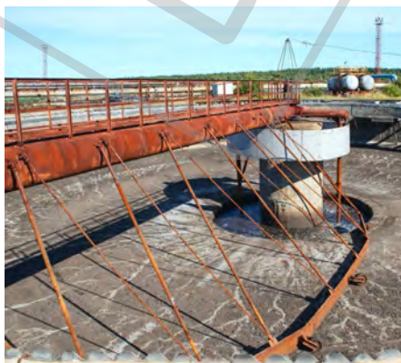
Figure 3.32 Flocculation results in the clumping together of suspended particles in waste water.
