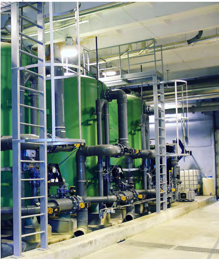
Figure 3.34 Chlorine and waste water tanks in a tertiary water treatment plant.
