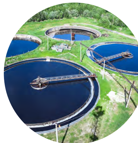
Figure 3.15 Sewage treatment involves sedimentation and flotation.
